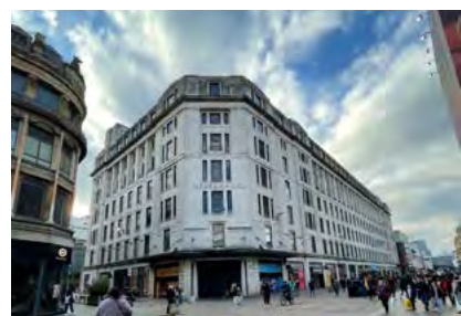
Former Debenhams building: conversion to grade A office has been consented
