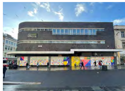
BHS Building: Current condition
