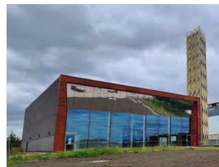
West Dunbartonshire Energy Centre, Clydebank
