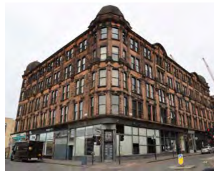
Wasps operated South Block, Osborne Street
