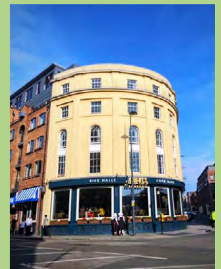
Casartelli Building before and after restoration
